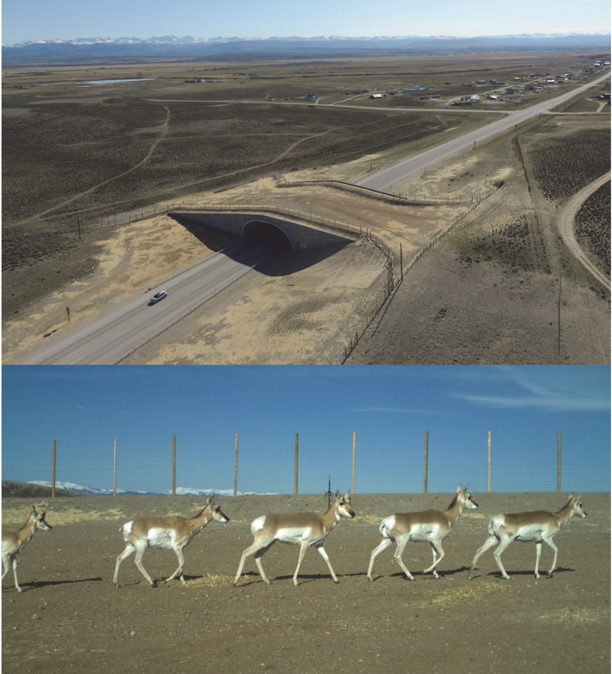
Figure 2. Aerial view of the Trapper's Point Overpass along US Highway 191 in western Wyoming, USA (top panel). Pronghorn crossing the overpass during fall migration 2013. Dirt berms provide visual barrier between animals and highway (bottom panel).
