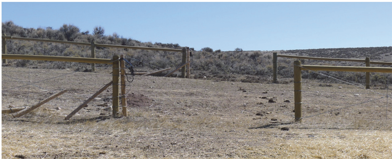
Figure 15. Fence gates at east approach to Boroff Hill Overpass.
